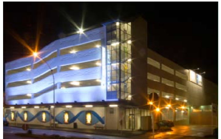
Knox Street Car Park, Hamilton
