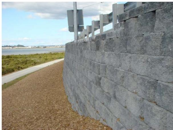
Firth retaining wall adjacent to MHX project using Diamond Pro bevelled retaining blocks in Rockface.
